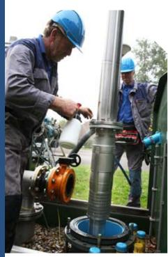
**Come together:** Vitens service technicians Drikus Geurtsen and Herman de Greeff install a new Grundfos SP submersible pump into a well at Loosdrecht. Below, De Greeff sprays the pump with chlorine to kill bacteria before lowering it. The seven Grundfos pumps better fit the flow demand of the well field, saving 21% energy.
